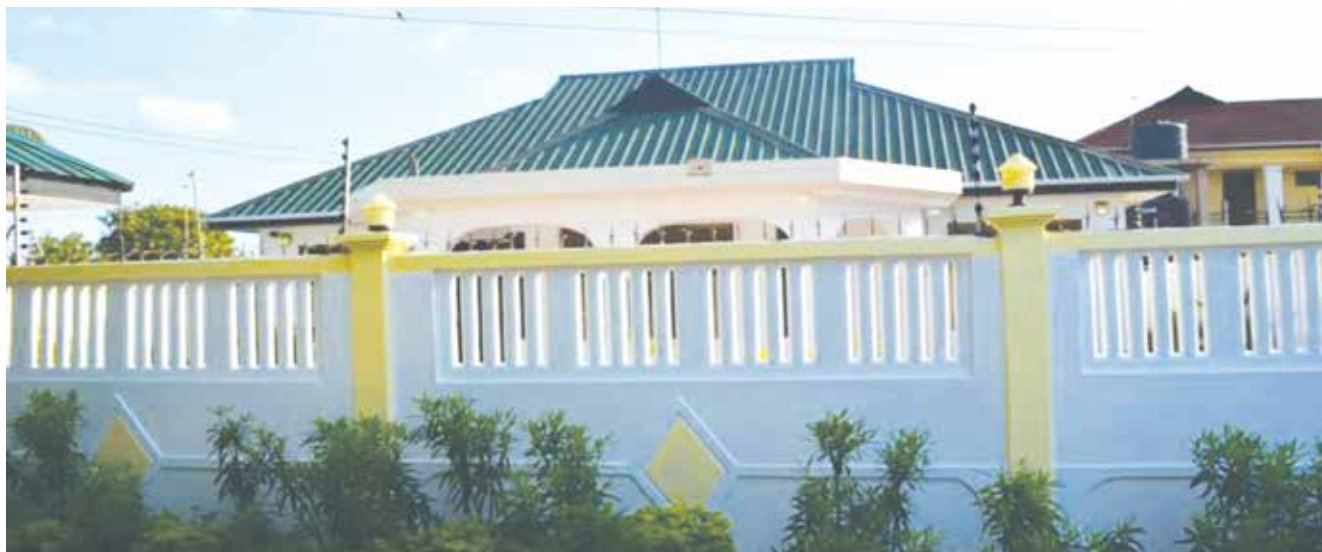
THRDC well protected office
